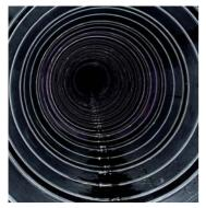
Sealing of a pressure pipe diameter 1800 with AMEX®-10 VARIO System
