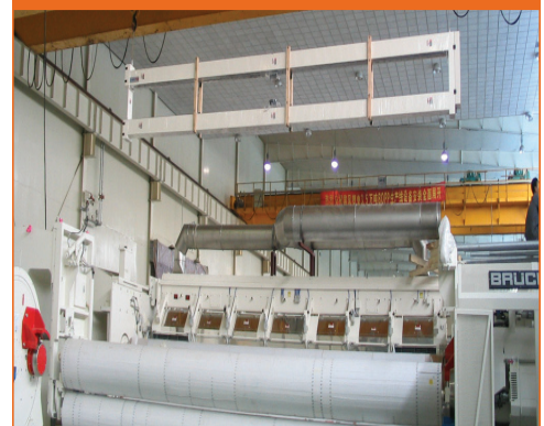
Installation of NDC scanner on 10.5 m wide BOPP line
