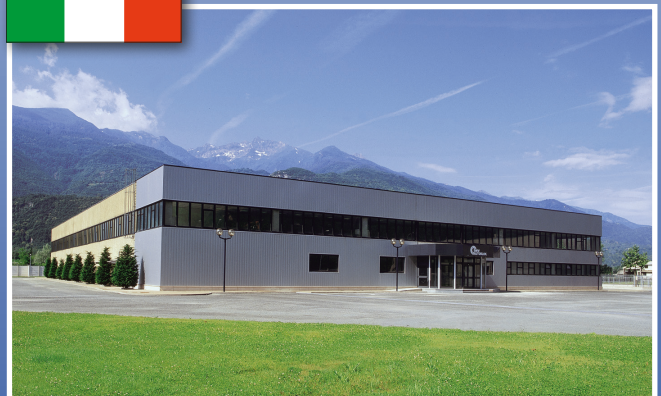
AUTOBLOK manufacturing plant Caprie-Torino
